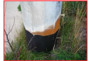
Pole Above Grade
