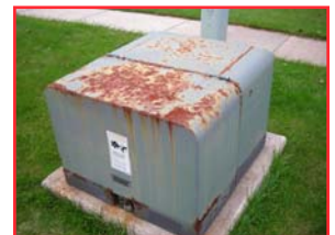
Padmounted Transformer
