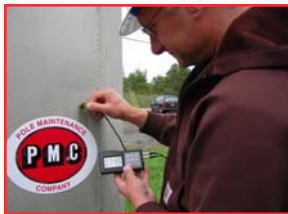
Ultrasonic Thickness Test
