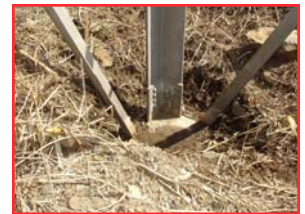
Tower at Groundline
